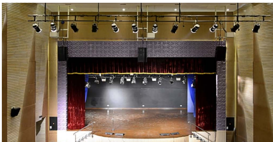
Centre, Right and Left speakers at Proscenium frame
